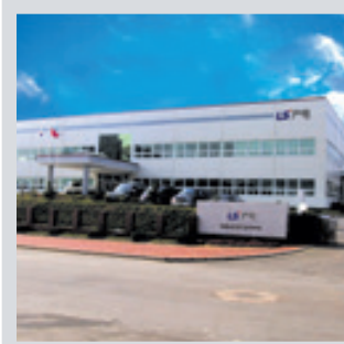
Dalian Plant (China)
