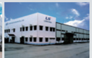
Hanoi factory (Vietnam) MV/LV switchgear, Mold TR
