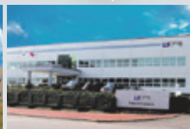
Dalian factory (China) MV/LV switchgear, MV contactor
